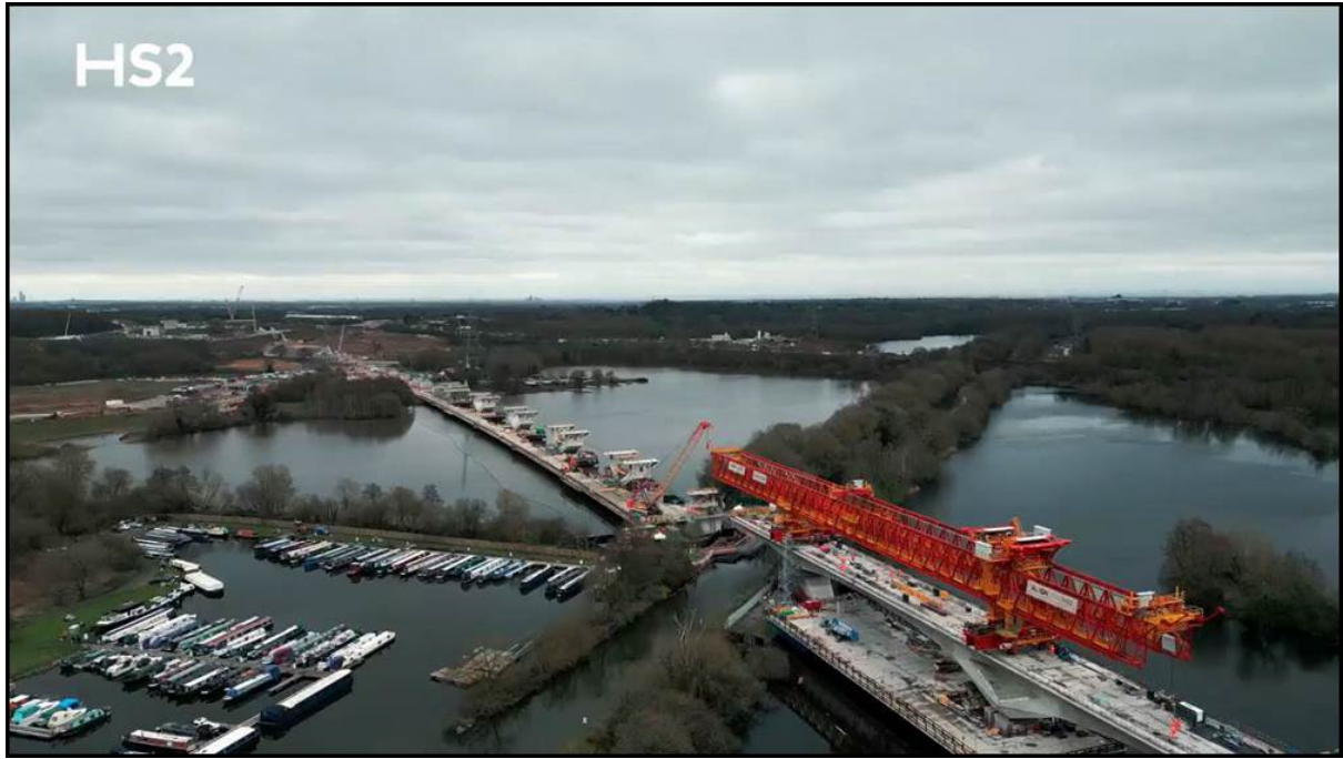
Photo below shows the remaining V-Piers in Harefield Lake No.2 (also shown in aerial photo above)
